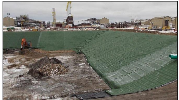
*Xtreme Armor System was installed atop a geosynthetic (top) and was secured with PDAs (middle). Even through cold and adverse conditions, the XAS saved the project substantially over a hard armor alternative (bottom).*
