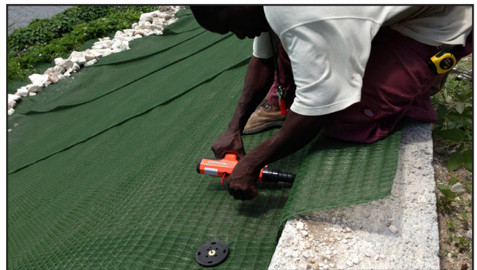
Project slope prior to installation (top), HPTRM placed on slope surface, pinned and anchored (middle). XAS fastened to the retaining wall to prevent flow from circumventing installation (bottom).
