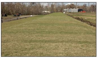
Meticulous installation of the Xtreme Armor System on the levee slope (top). The HPTRM was installed with PDAs along a high-impact curved levee face (middle). Sod installed over the XAS was established and ready for maintenance activities within 60 days of installation (bottom).
