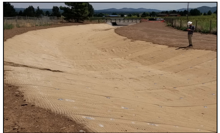
Percussion driven anchors were installed at 4 ft intervals across the HPTRM, with twist pins installed intermittently (left). The finished install of the ARVS design resulted in a low-impact design in the drainage channel (right).
