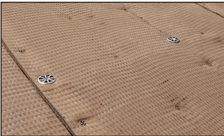
Percussion driven anchors were installed at 4 ft intervals across the HPTRM, with twist pins installed intermittently (left). The finished install of the ARVS design resulted in a low-impact design in the drainage channel (right).
