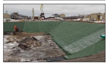
Xtreme Armor System was installed atop a geosynthetic (top) and was secured with PDAs (middle). Even through cold and adverse conditions, the XAS saved the project substantially over a hard armor alternative (bottom).
