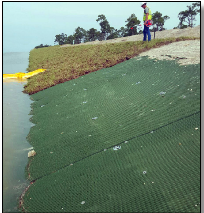
Armored shoreline with vegetation in place and prior to sod.
