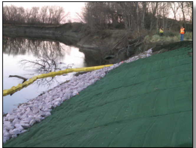
Armored shoreline with riprap toe prior to vegetation establishment.
