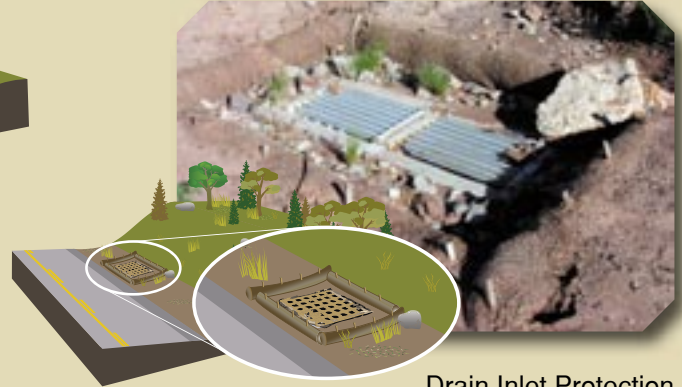
Drain Inlet Protection
